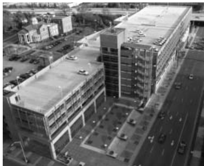
The 4th Street Parking Deck as of January 2006
